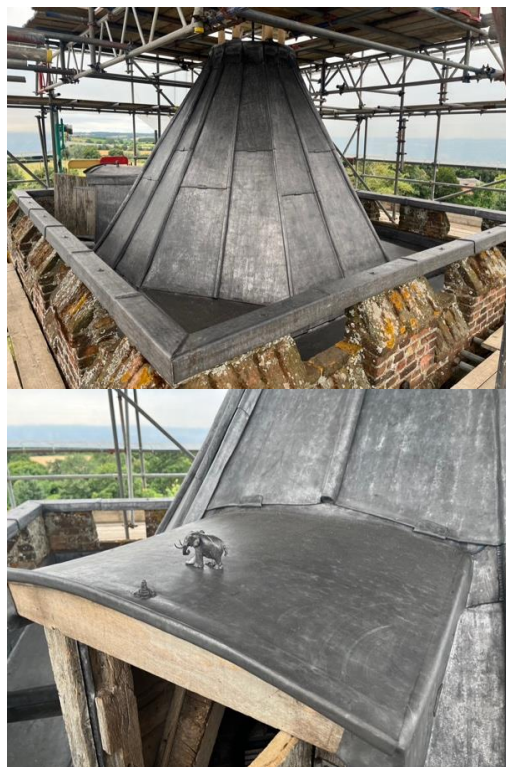
The new Tower roof – Spot the elephant!
