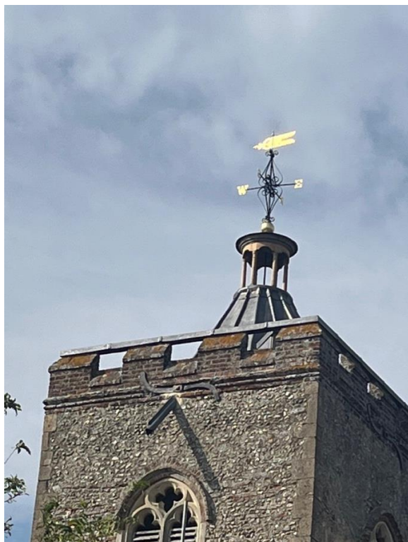
Sparkling new Tower roof & Cupola
