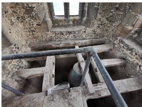
Troston: Re-hung on a new steel frame
